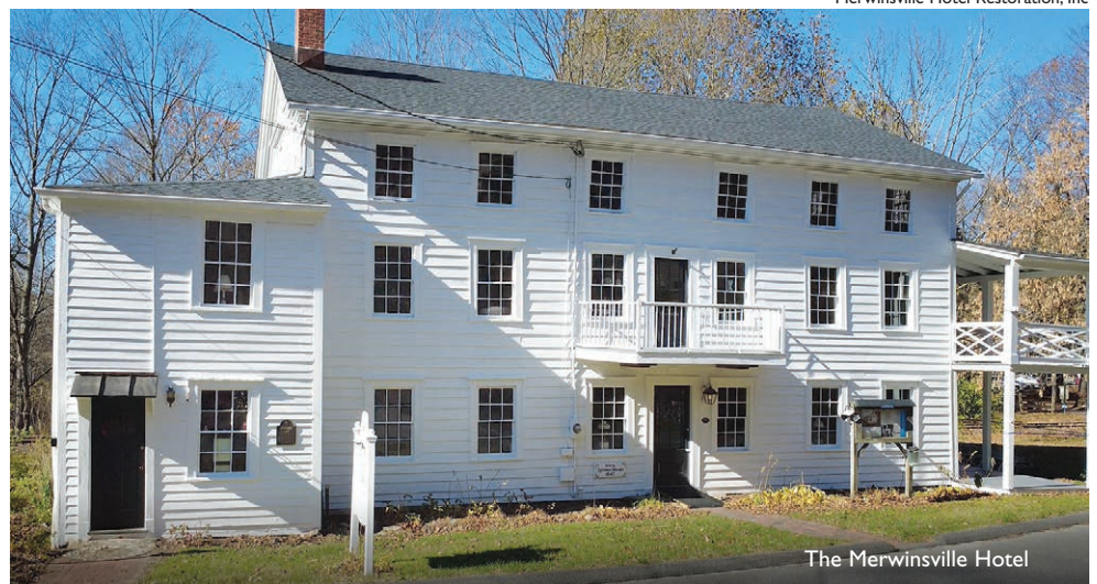
Merwinsville Hotel Restoration, Inc
