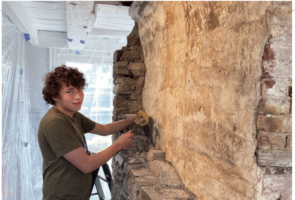
Jack Lovejoy restoring historic masonry
