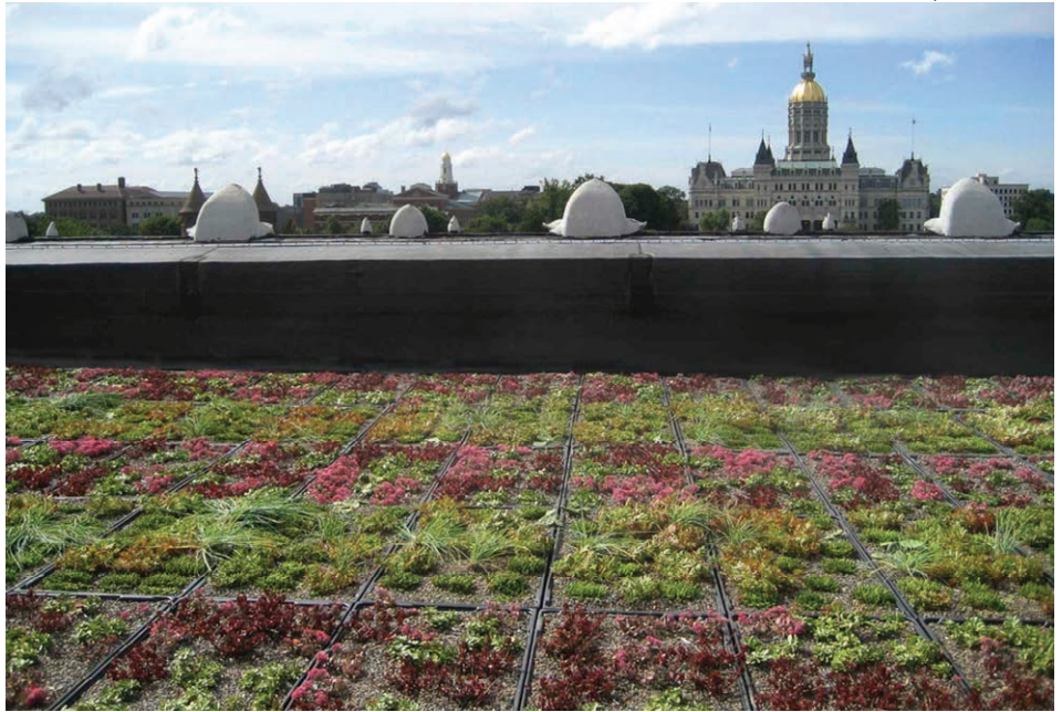
Green roof at the Betty Ruth and Milton B. Hollander Foundation Center.
