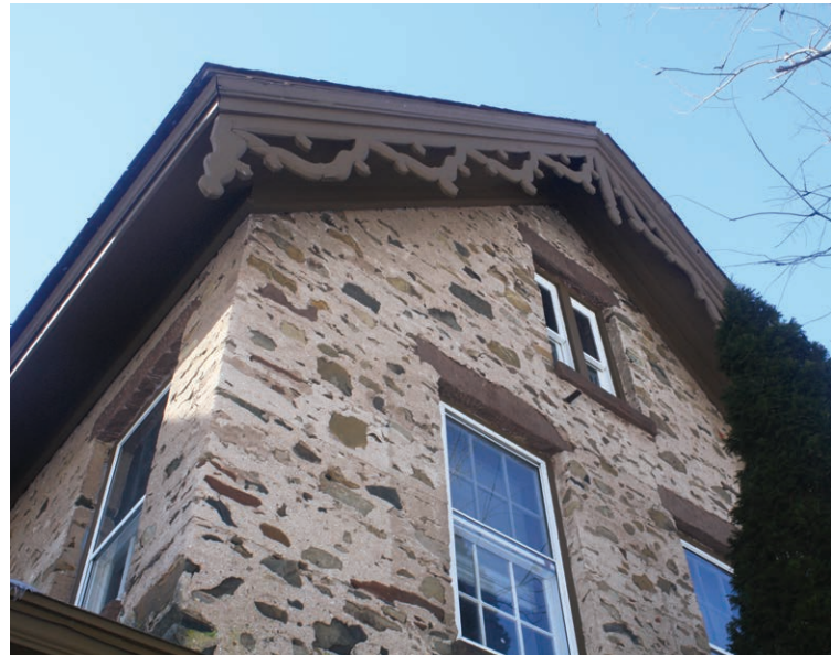
BELOW: Stonehouse: detail of concrete construction showing horizontal marks left by the forms.
